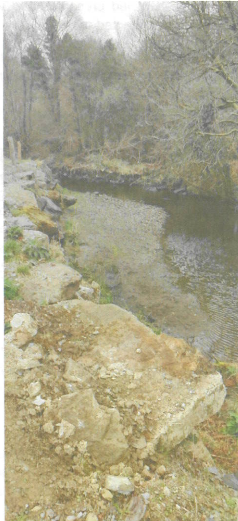
Figure 5 Rock armour adjoining the proposed development area with some recolonization occurring. Deeper glide section of the Bandon River also evident.
